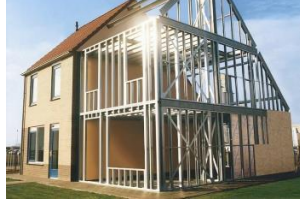
Figure 2. Cold-formed steel structure system of a residence employing a light steel framing system (LSF) [1].
