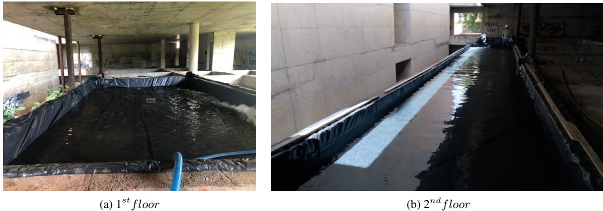
Figure 4. Loading test of the first and second floor.
