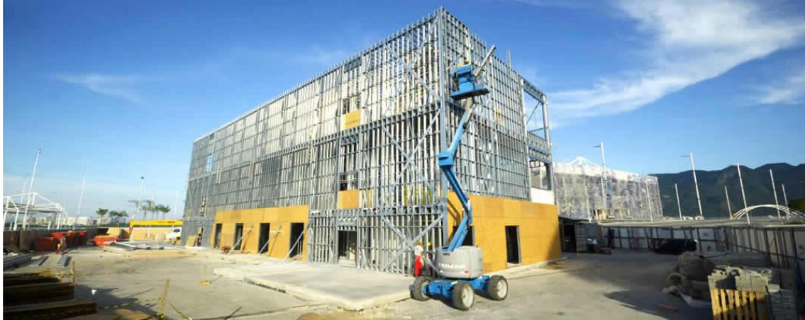
Figure 1 –Light steel frame using cold-formed steel members [2].
