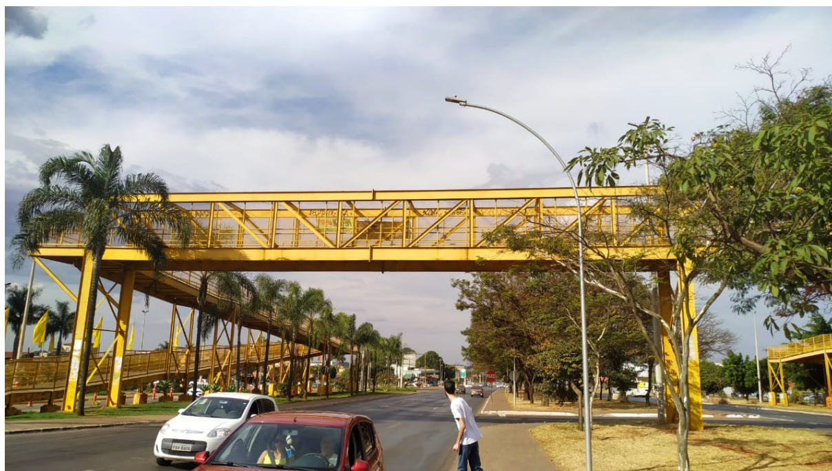
Figure 1. Front view of the steel bridge located in Brasilia, Brazil.
