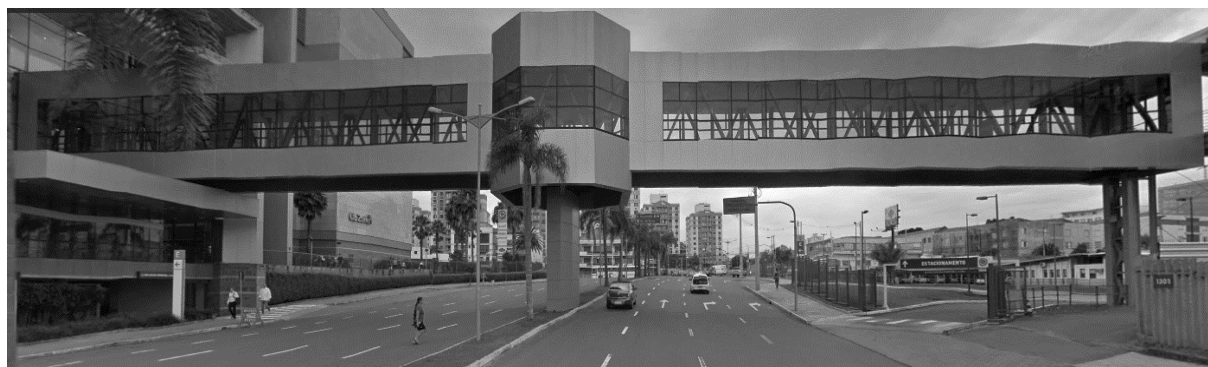
Figure 1. Bourbon Wallig Footbridge
