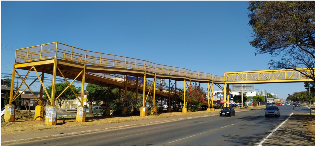
Figure 1. Front view of the steel bridge located in Brasília, Brazil.
