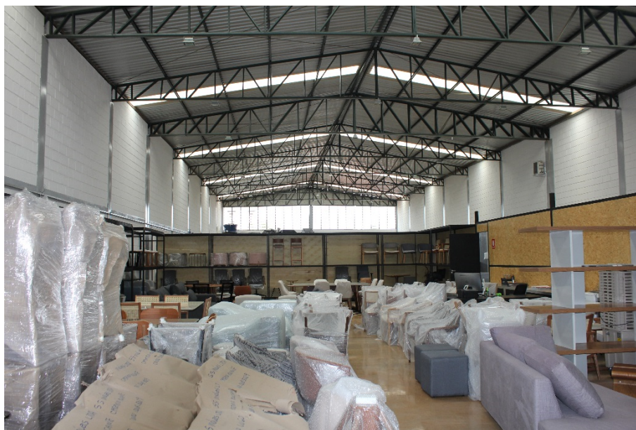
Figure 1. Interior view of the steel industrial warehouse located in Brasilia, Brazil.
