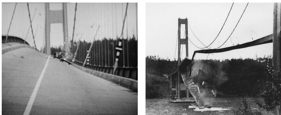
Figure 5. Dynamic instability: resonance in Tacoma Narrows Bridge (Tacoma – WA, 1940)
