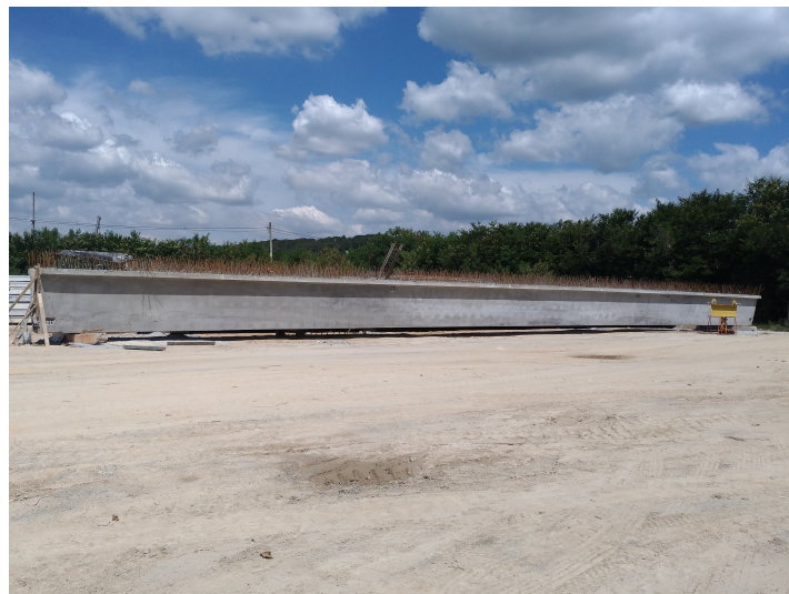
Figure 2. Prestressed concrete beam in storage
