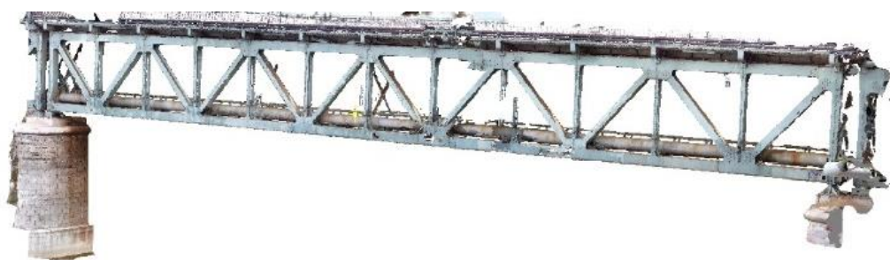
Figure 5. Façade of steel truss bridge
