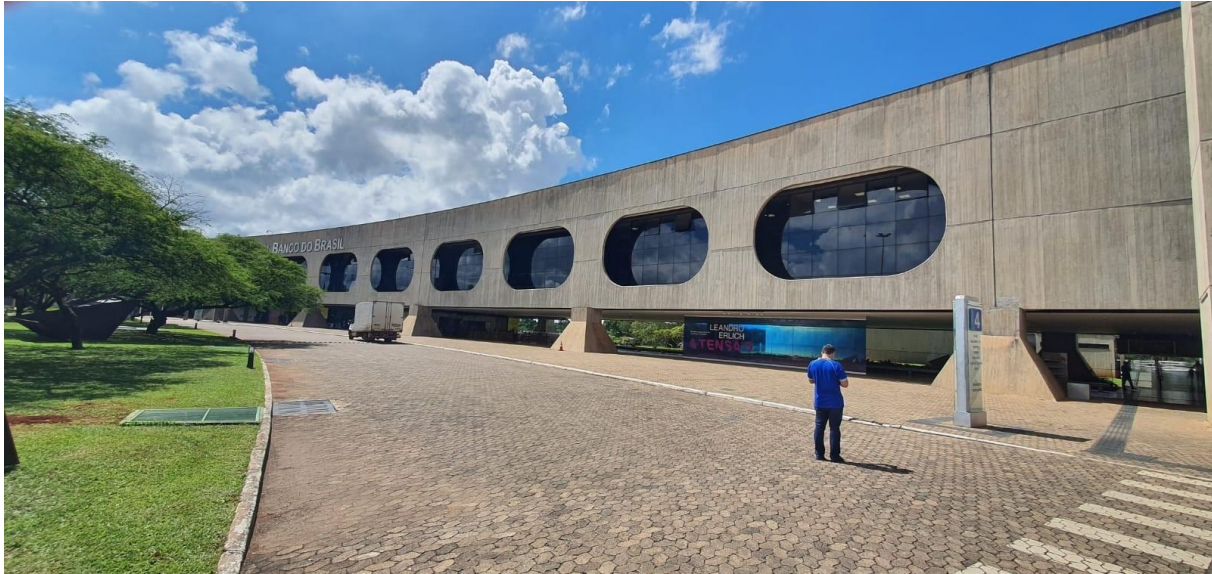
Figure 1. View of the façade of the Tancredo Neves building, showing openings in the external wall and the columns in the form of a pyramid trunk. Author's photo
