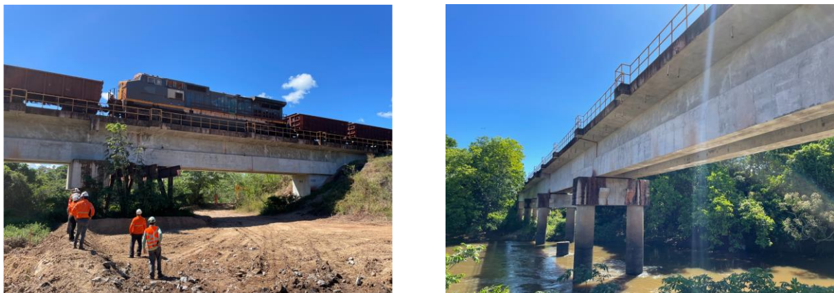
Figure 1. Reinforced concrete railway bridge employed as a case study
