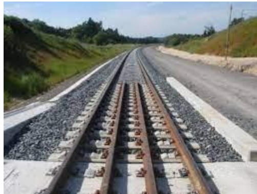
Figure 1 - Ballasted-slab track transition zone
