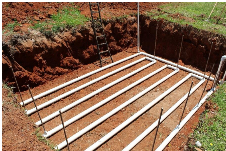
Figure 1. The experimental model of the EAHE built at UTFPR – Ponta Grossa
