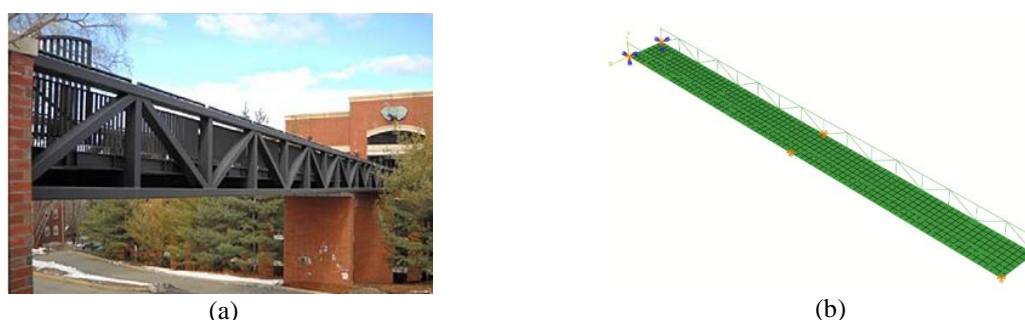
Figure 1. View of the Dowling Hall Pedestrian Footbridge (a) and the FE Model created in Abaqus (b)
